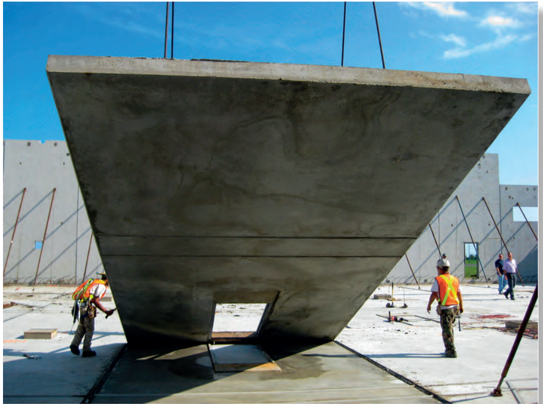
Tilt-up reinforced concrete wall panel
