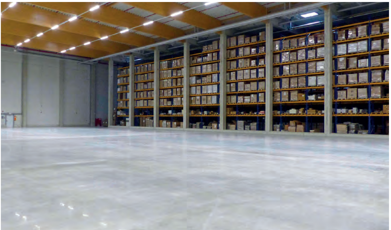
Concrete warehouse, Becosan concrete floor
