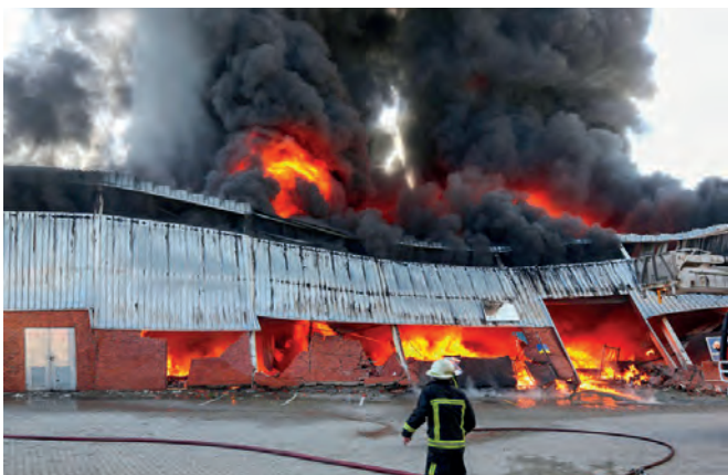
Steel structures offer limited fire structural integrity
